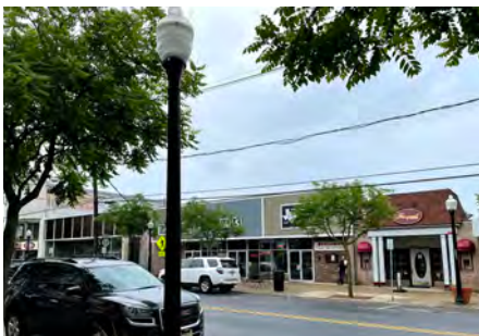
Existing 1-Story Buildings
